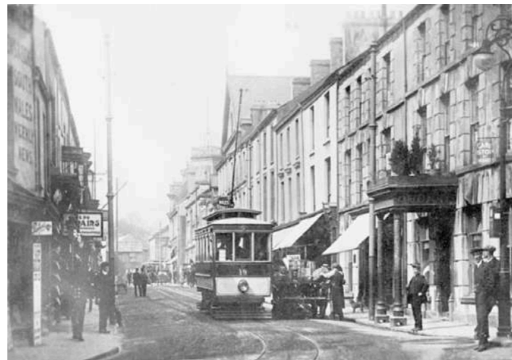
Canon Street. Trams came to Aberdare in 1913 & ceased running in 1935.
